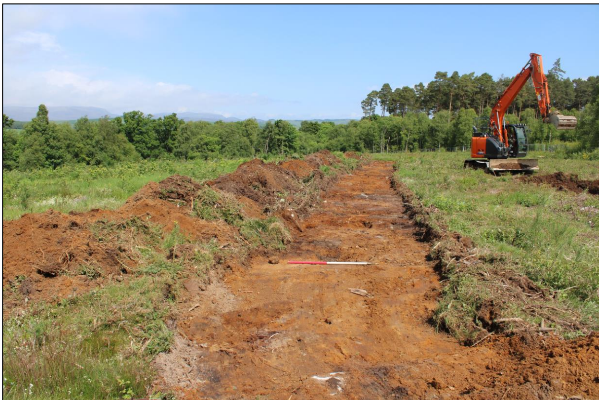
Figure 10: Post Ex of Trench 11, North facing, Photo No.1262
